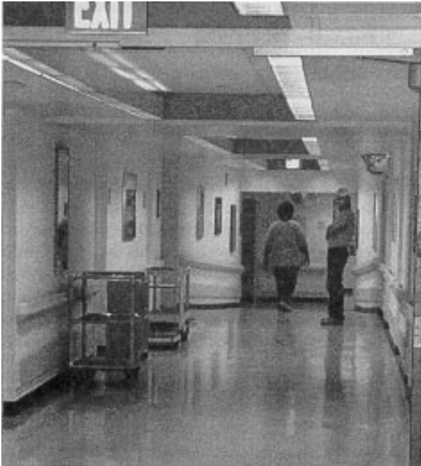
Figure 7-3—Corridor lighting, using linear fixtures, after remodeling
